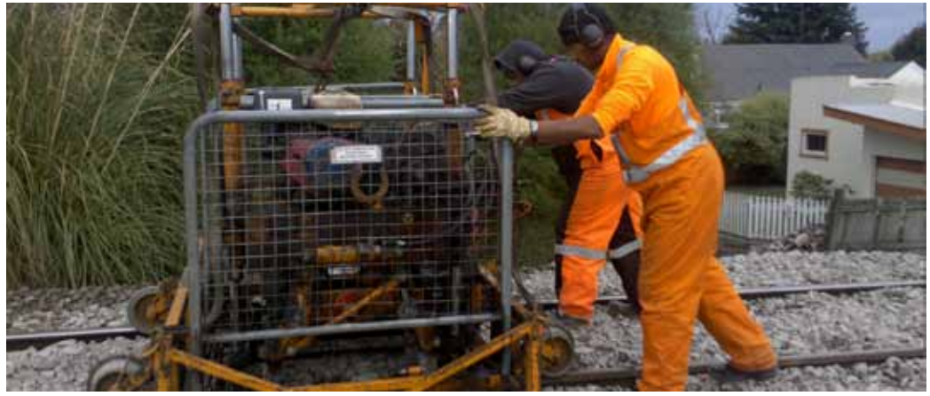
Network staff adjusting track near Kaiapoi using a mini tamper on Sunday.
