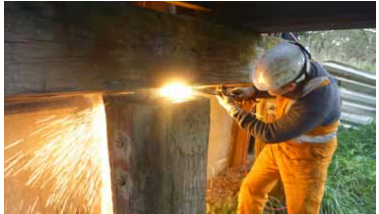
Brodie Neville, Leading Hand and Acting Structures Inspector, cutting the boltwork on the failed Number 1 end of Bridge 18 yesterday.
